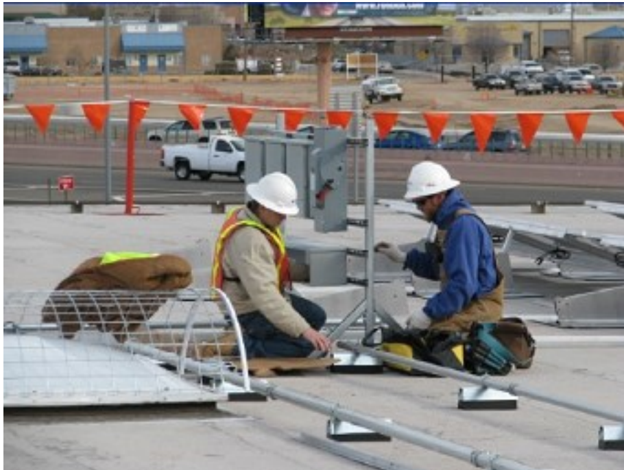
Figure 10 – Example of warning line
