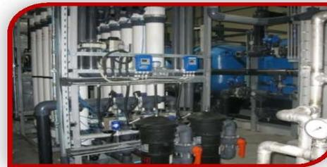
The process design was a challenge with respect to the high overall design recovery requirement of 80% and 100% of NH<sub>3</sub> removal necessary to protect the copper cooling systems tubes from corrosion.
