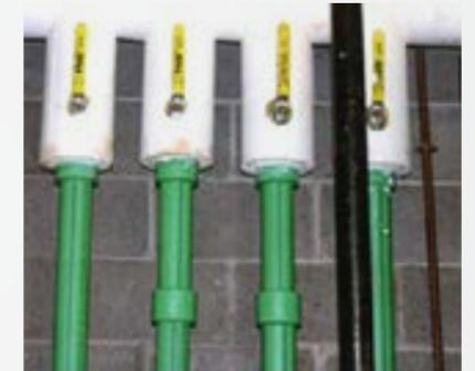
Thermal Insulation of PPR tubes at roof Plumbing
