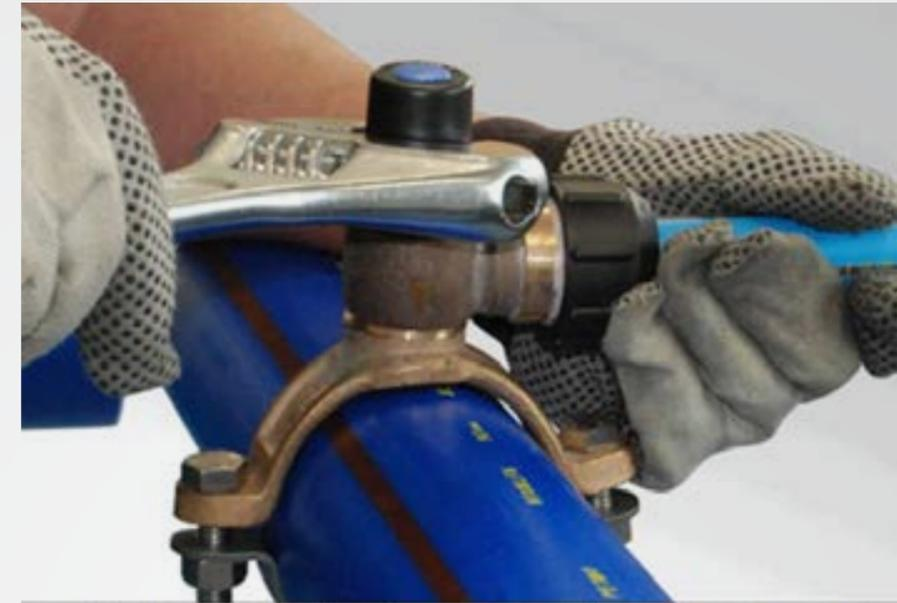
Gun Metal Ferrule tapping from compound internal water net work to the corresponding villa or other
